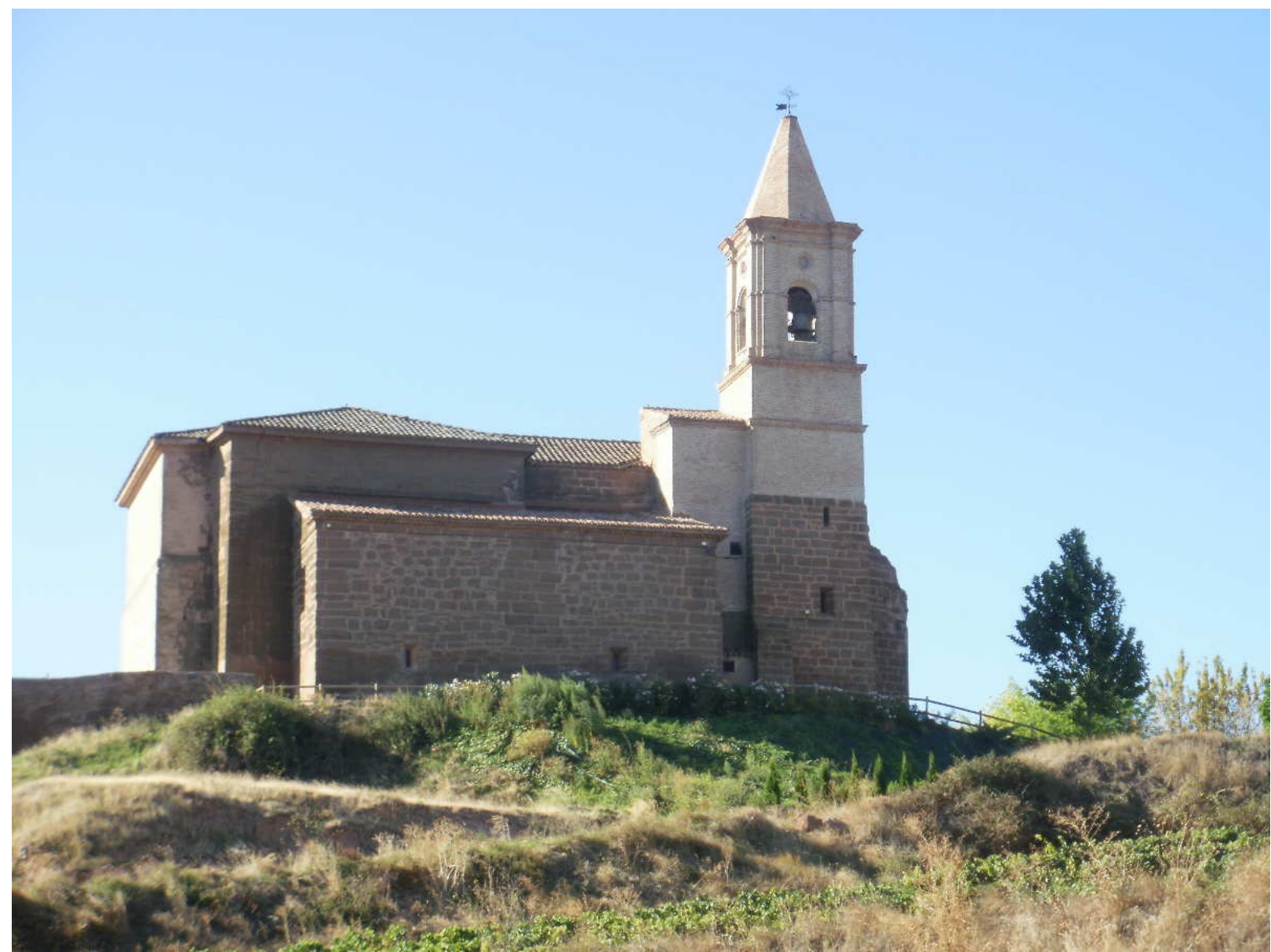
San Saturnino of on the outskirts of Ventosa
