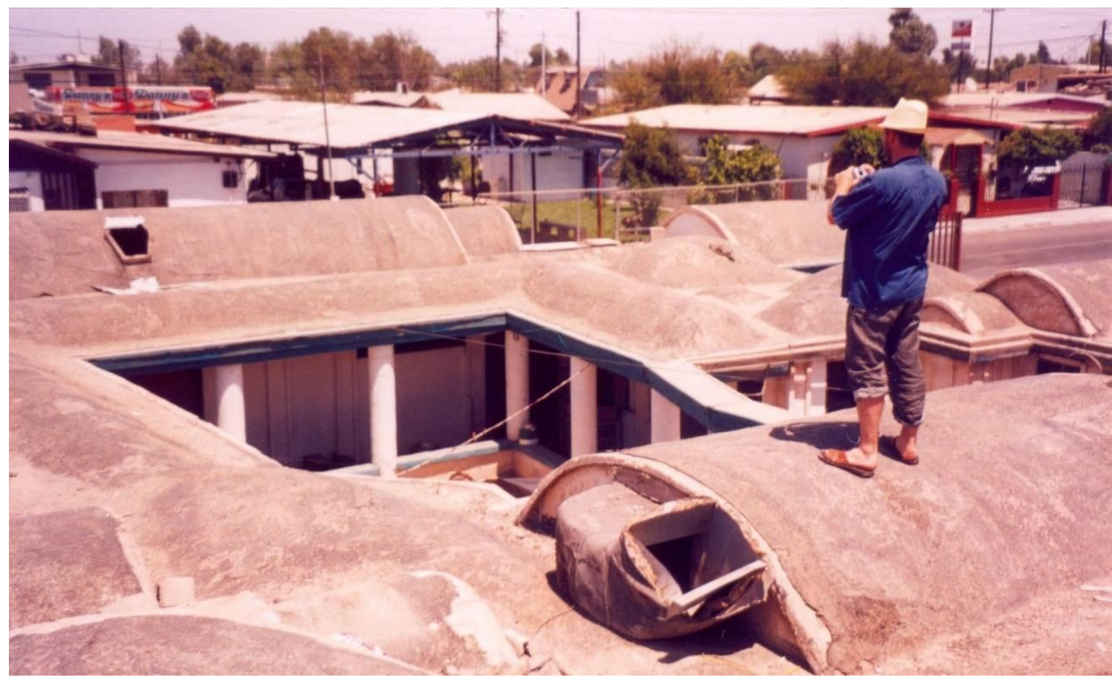
Construction of Mexicali Project (Photo courtesy of Dr. Robles)
