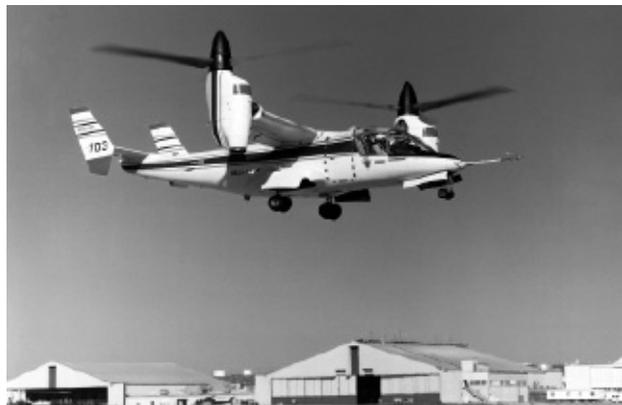
*The NASA/Army/Bell XV-15 Tilt Rotor Research Aircraft in flight. NASA.*
