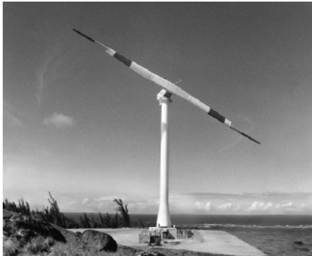
*DOE-NASA Mod-5B 3.2-megawatt wind turbine, Oahu, HI. NASA.*
