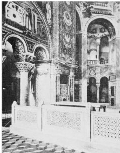
FROM THE INTERIOR OF SAN VITALE, RAVENNA SHOWING THE “IMPOST” ABOVE COLUMN, AND DECORATION.
