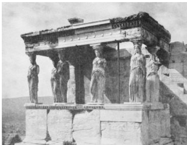
PORTICO OF THE CARYATIDES. ERECHTHEION IONIC ARCHITRAVE AND CORNICE; NO FRIEZE. P. 141
