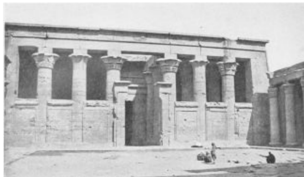
TEMPLE OF EDFOU ENTRANCE TO HYPOSTYLE HALL. METHOD OF ADMITTING LIGHT IN PTOLEMAIC PERIOD. P. 54
