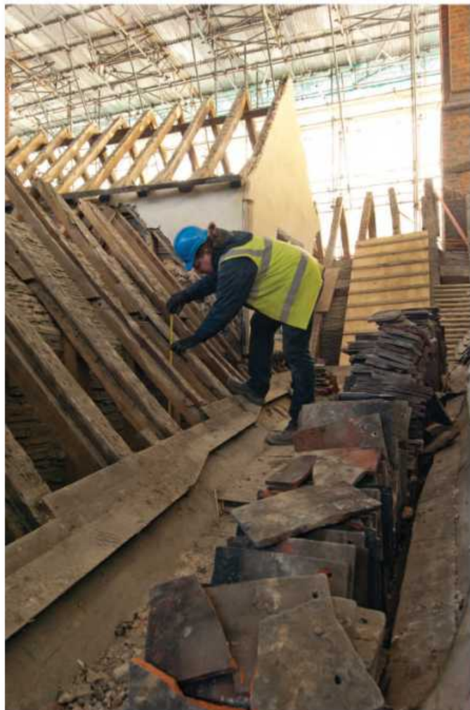
The examination of roof timbers at Knole House has revealed that much of the wood was recycled from at least five earlier roofs, possibly reflecting a financial need to save money.
