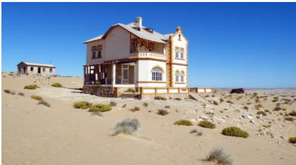
The restored Manager's House: – Kolmanskop.
