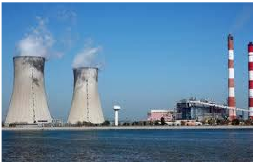
Plate 8.1. Guru Hargobind Thermal Plant, India. Source: http://www.treehugger.com/living/
