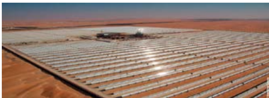
Plate 7.1. Concentrated solar power plant at Shams in the UAE Photo from [4]
