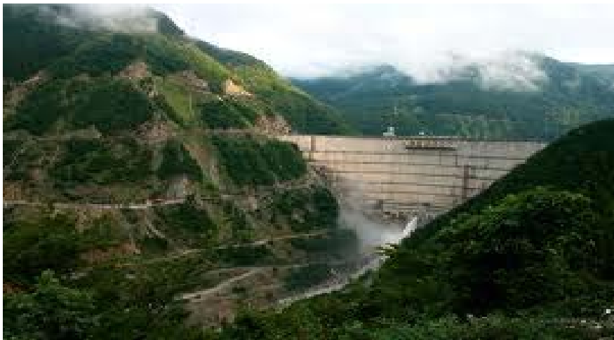
Plate 11.2. Inguri Dam in Georgia. Image sourced from [12].
